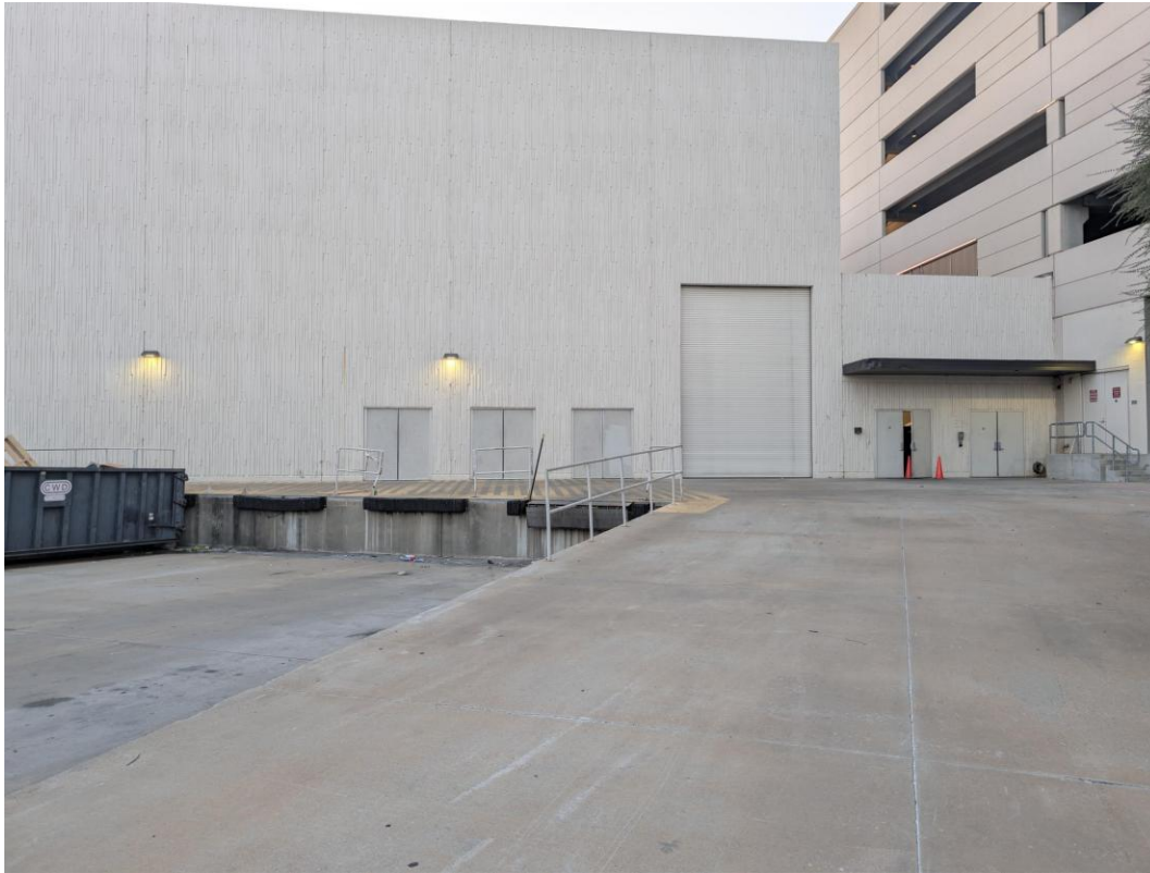
Loading Dock Area — Center roll-up door provides direct access to Terrell Hall. Entry door with orange cone (right side) is the Starlight Ballroom entrance — press intercom to be buzzed in.
